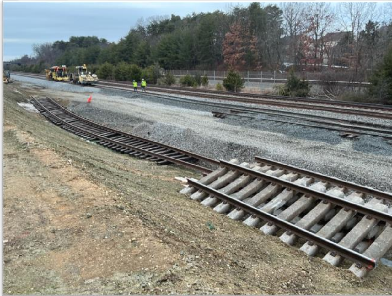
Track removal at Future CP Beltway
