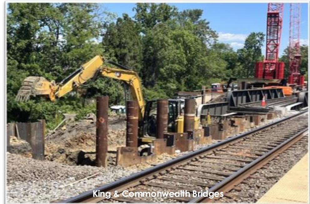
Long Bridge South Package
