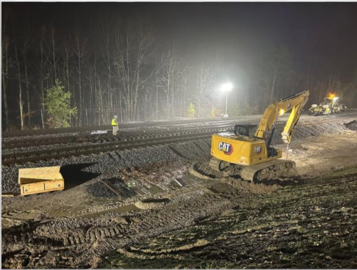
Turnout panel installation at Future CP Beltway
