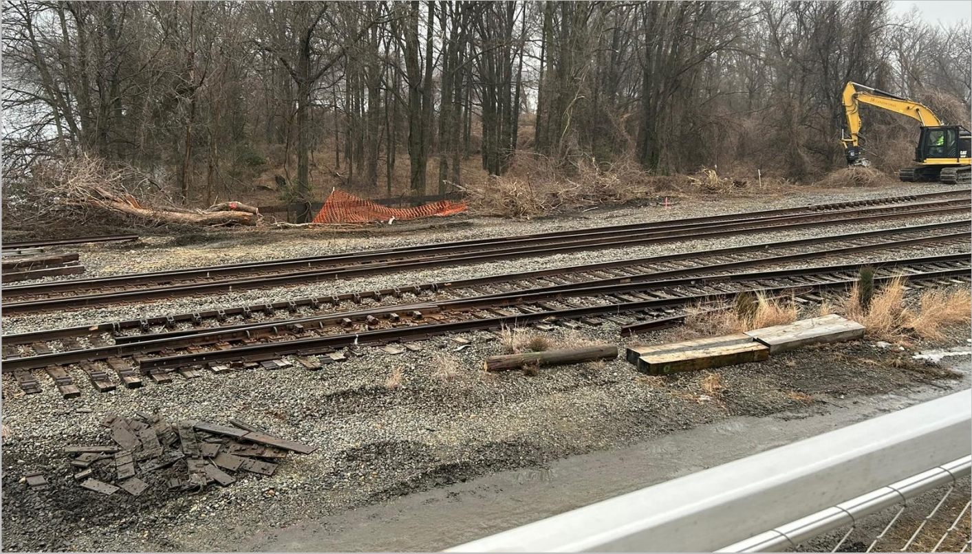
Clearing & grubbing at Long Bridge Aquatic Center
