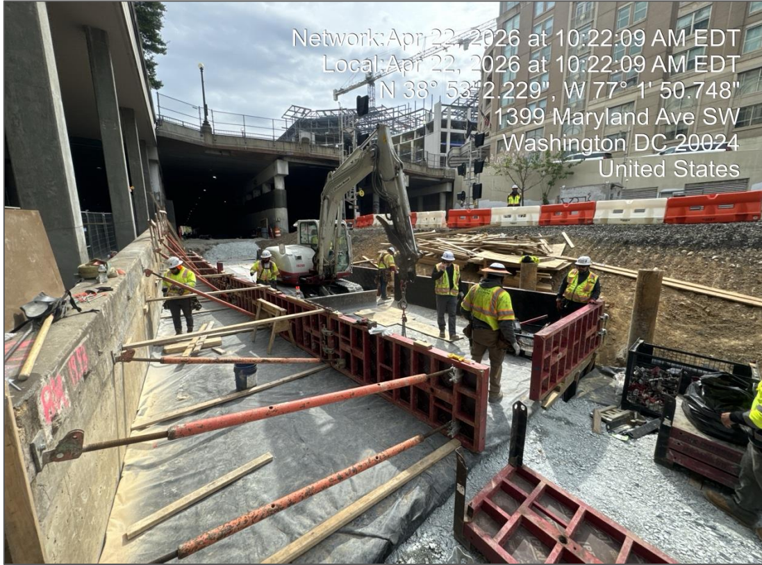
Near Maryland Ave. overbuild
