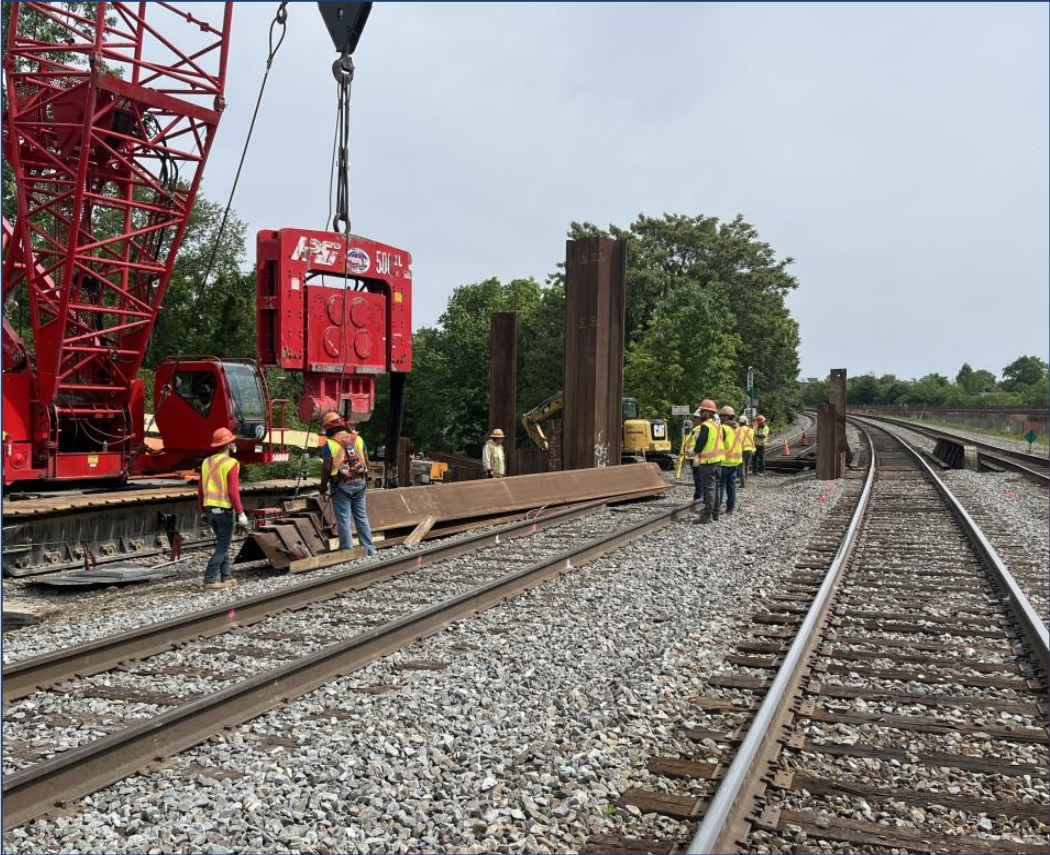
Vibrating sheet pile driver on Track 3
