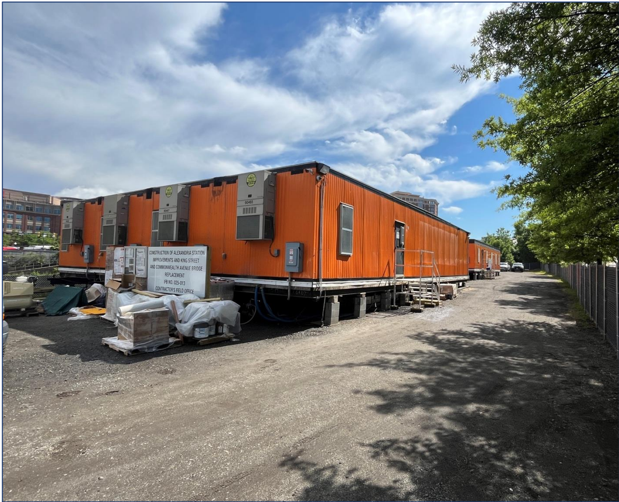
Field office installation
