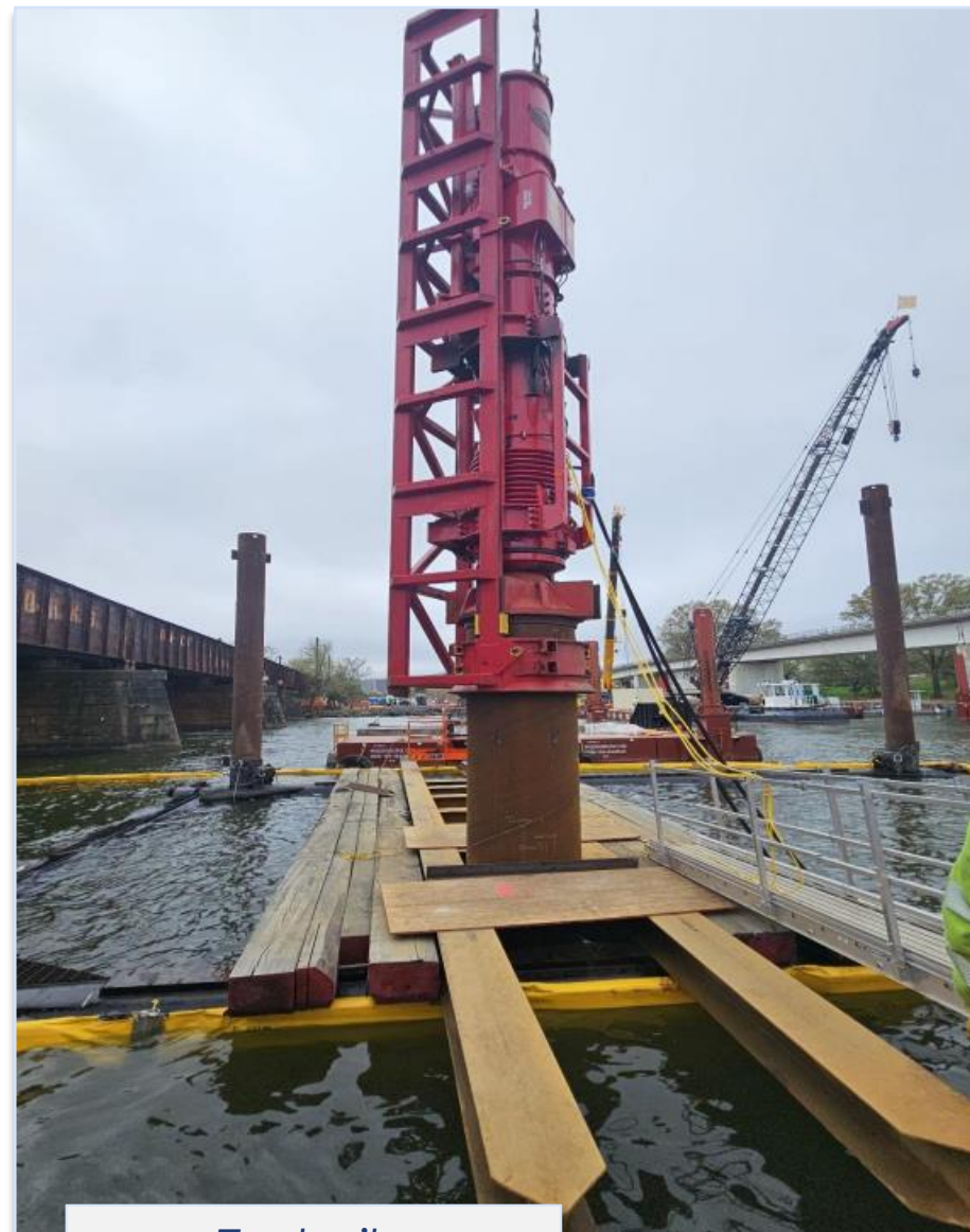
Test pile installation in the Potomac River
