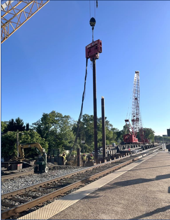
Pile driving guide beams
