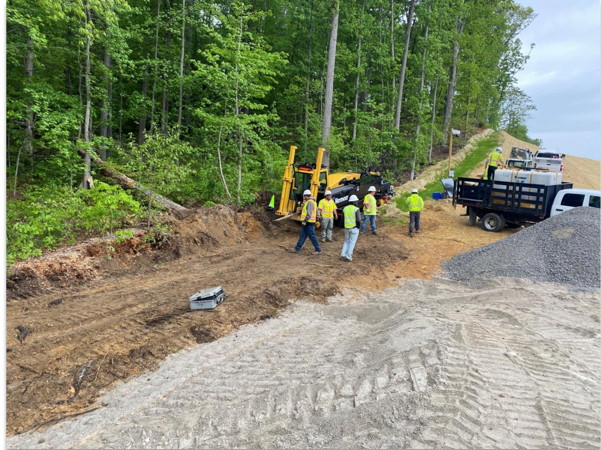
Fiber optic utility relocations
