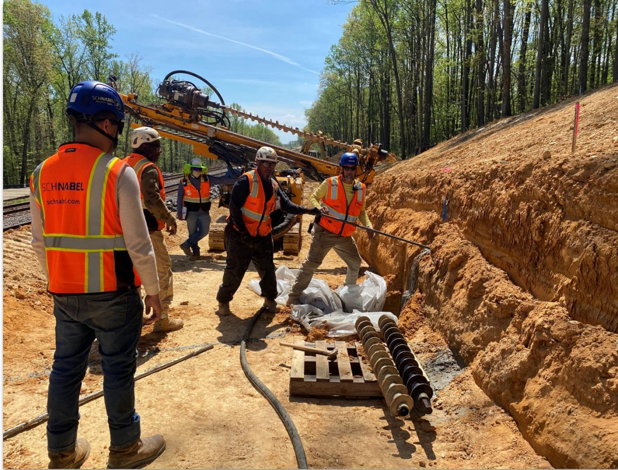
Soil nail installation for retaining walls
