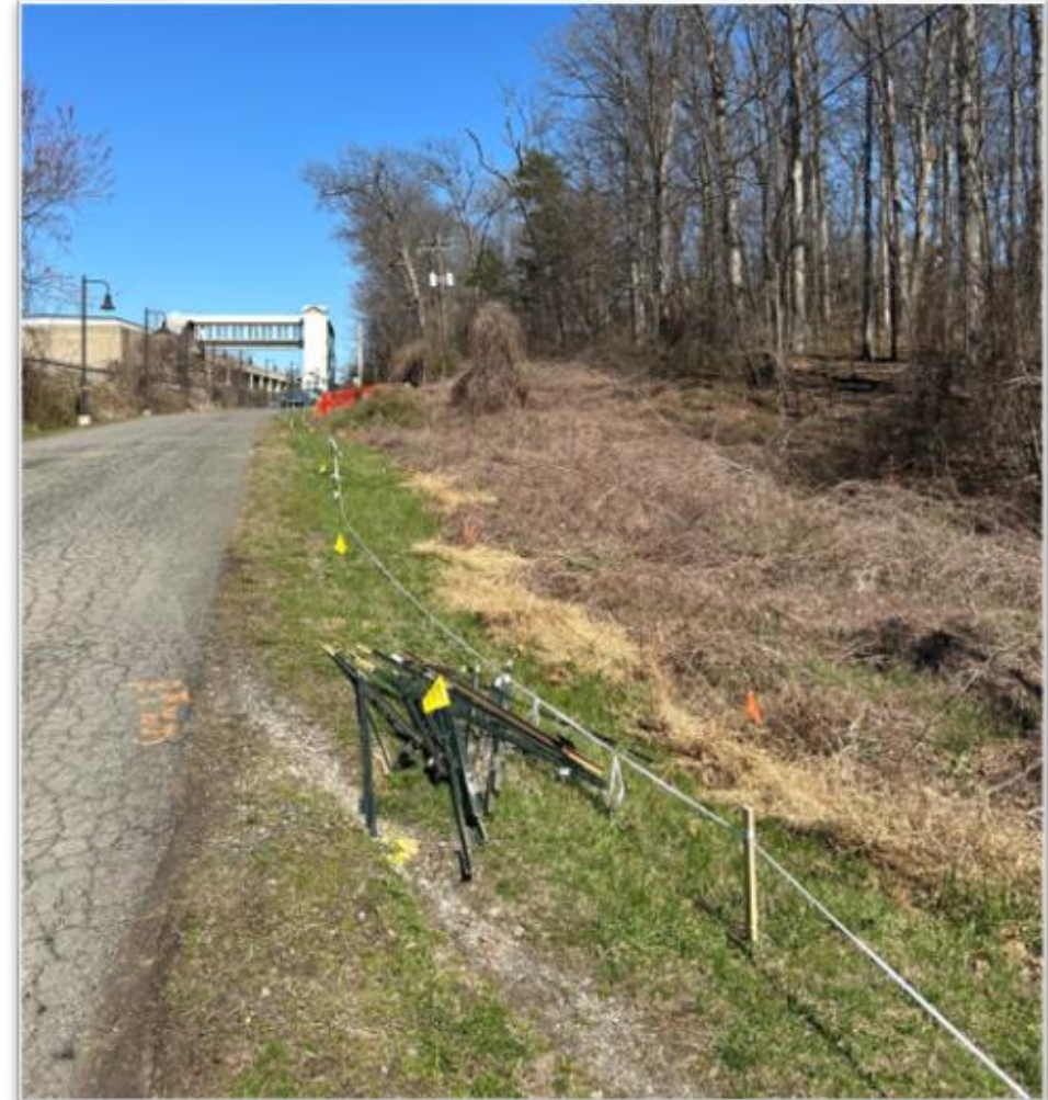
Tree & brush clearing for utility relocations at Barry Road
