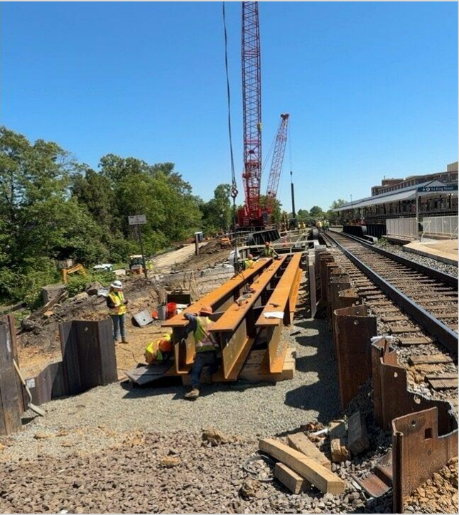
Track 3 jump span beam installation
