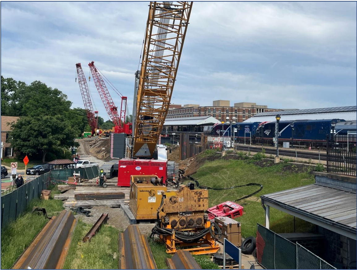
Cranes delivered on site
