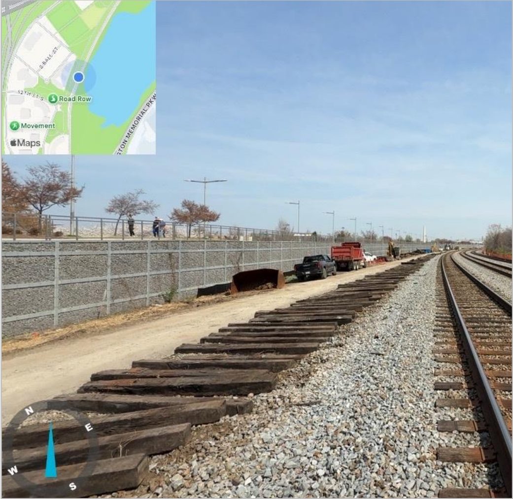
Out-of-service track demolition at CP RO
